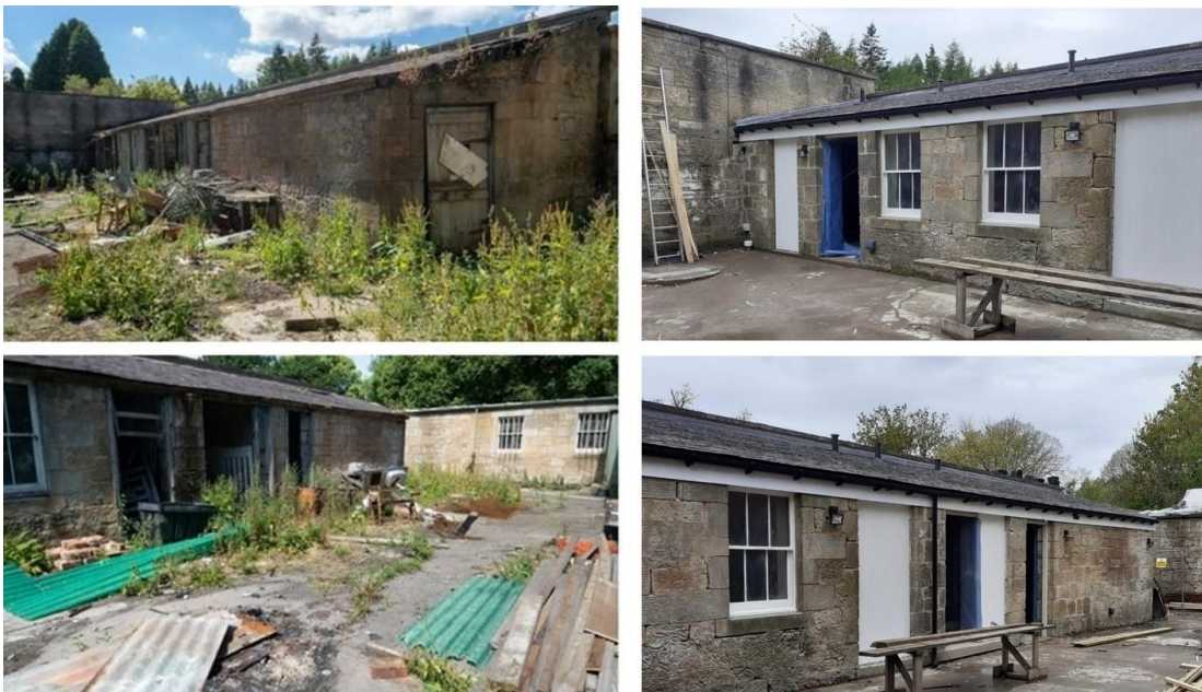
Courtyard outbuildings refurbished mainly through the lockdown period.
